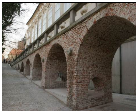
Fig. 7. The drying brickwork after removing the old plaster.
