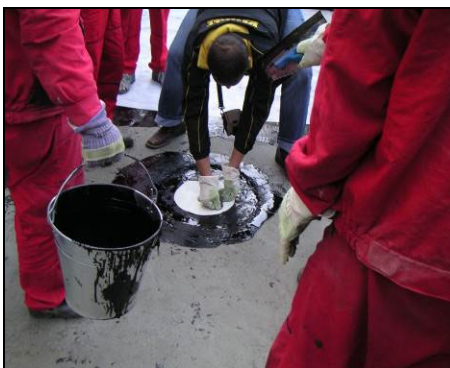
Fig. 11. The working on the first layer of hot asphalt waterproofing membrane Bakor 770, a rubber sheet around the connection of drain pipe on the right side.
