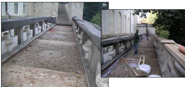
Fig. 9. The situation after the installation of new drains pipes with electrical heating, the installation of power cables on the right side.
