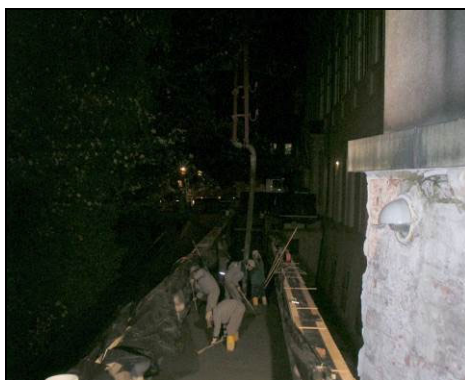
Fig. 10. The night work with concrete and new reinforced concrete deck slab modified silica fume.
