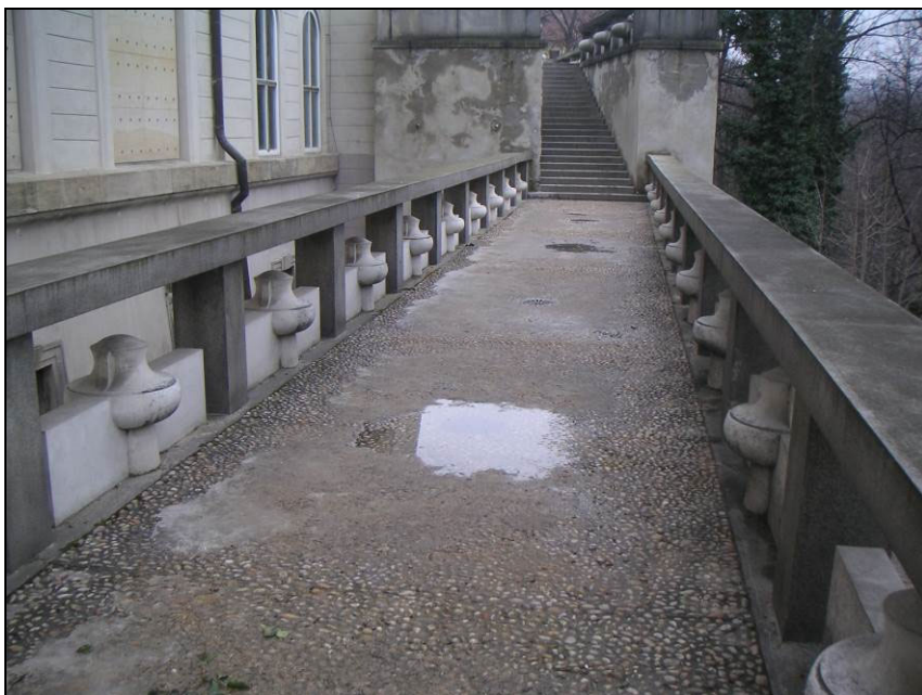
Fig. 4. Water from melting snow and ice on deck in 2004.
