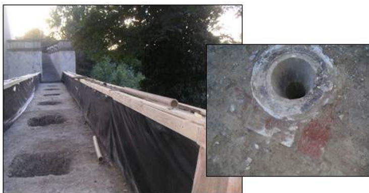
Fig. 8. The state after the destruction and demolition of the existing bridge deck drainage, original design end of the drain pipe on a right side.
