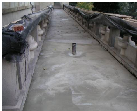
Fig. 10. The night work with concrete and new reinforced concrete deck slab modified silica fume.
