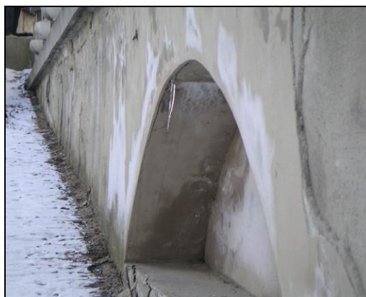
Fig. 3. A closer look at the the state of lower construction - icicle on a significant crack in 2004.
