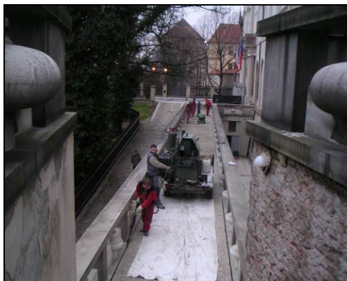
Fig. 15. The hot asphalt modified grout joints by Bakor 513 in November 2006.
