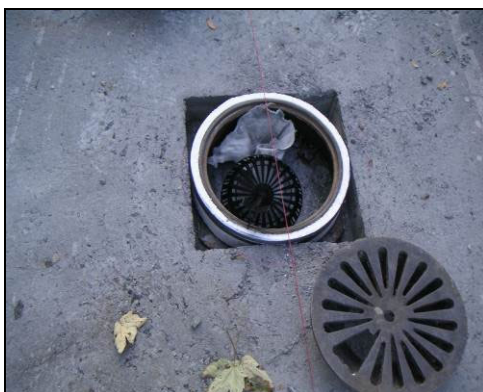
Fig. 13. To refit original gullies in 2006.
