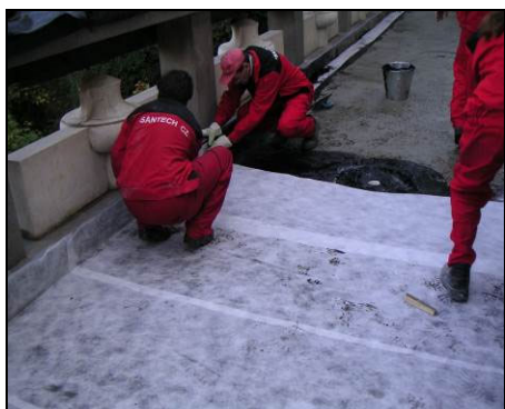
Fig. 11. The working on the first layer of hot asphalt waterproofing membrane Bakor 770, a rubber sheet around the connection of drain pipe on the right side.
