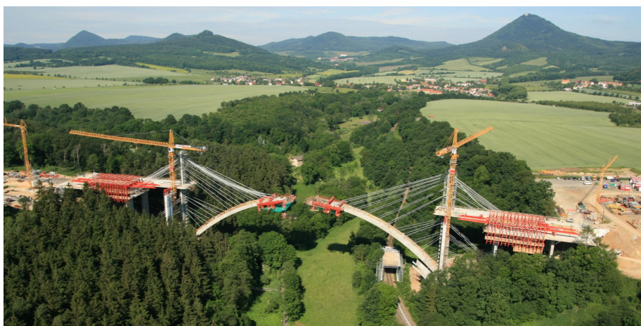
Fig. 4. Progressing cantilever construction.
