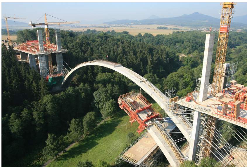
Fig. 5. Free cantilevering of the second arch.
