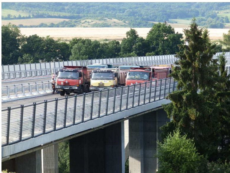
Fig. 6. Load test.
