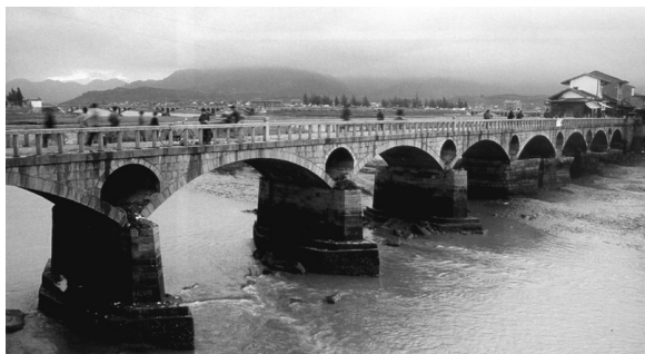
Figure 1: Jiang-kou Bridge in Putian, Fujian Province.
