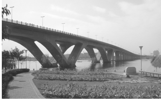
Figure 2: Yuxizhou Ming River Bridge in Fuzhou.
