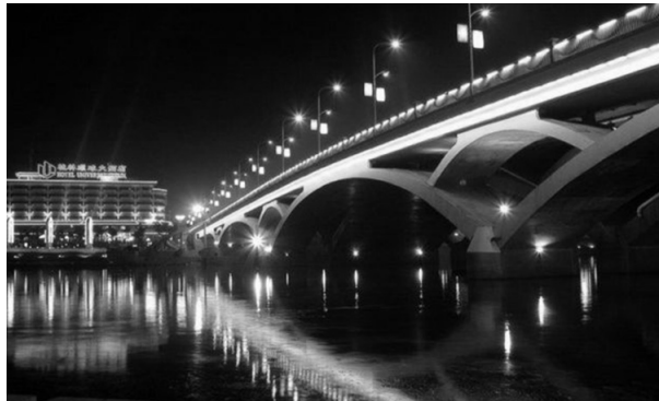
Figure 3: Jiefang Bridge in Guilin.
