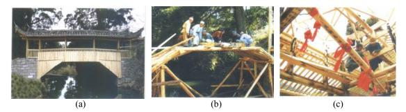
Figure 8: Shijin Bridge: (a) The Shiijin Bridge, (b) Install the main arch rib, (c)Raising of the ridgepole
