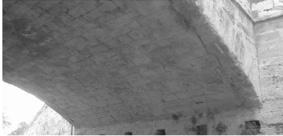
Figure 1. Damage in the stone in the end bridge bays.
