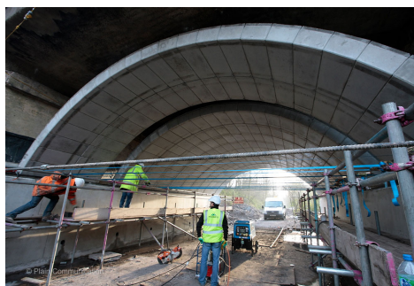
c) Sliding FlexiArch units along sill beams
