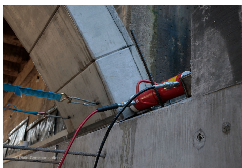
b) Hydraulic jacking system utilised.
