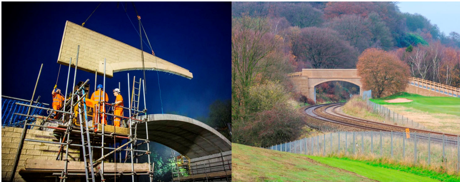
c) Installing spandrel wall
