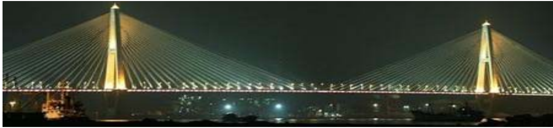
Qingzhou Min River Bridge
