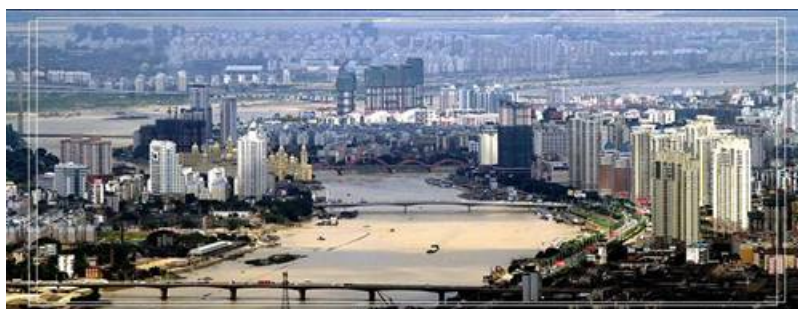
Bridges in Min River
