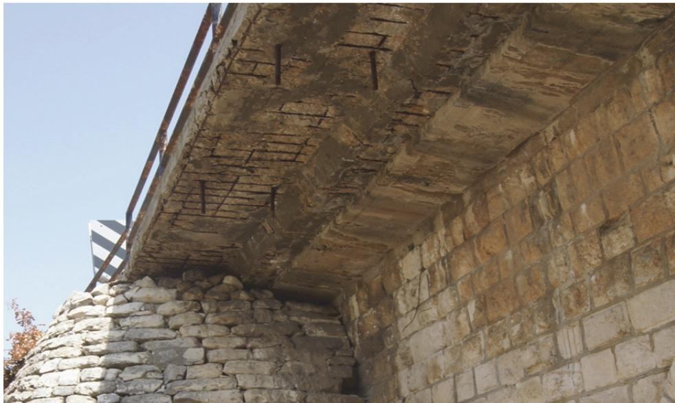
Figure 3: The poor condition of the bridge widening decks
