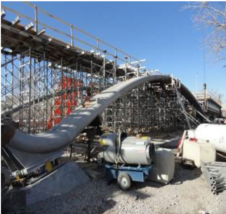
Fig. 8. Completed centre arches.
