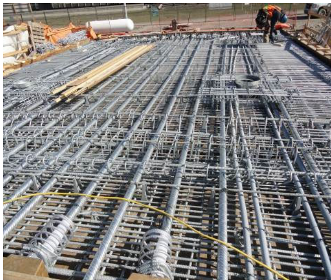
Fig. 10. Deck reinforcing bars and PT ducts.
