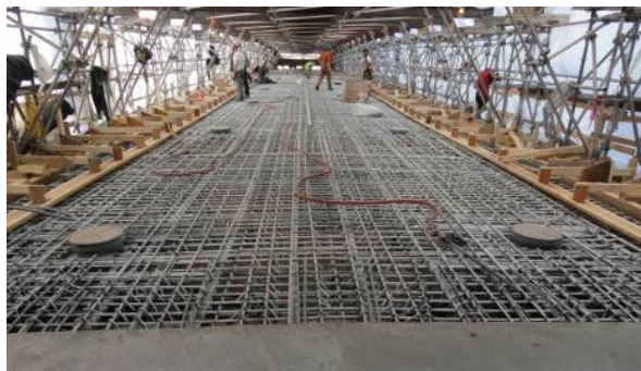
Fig. 18. Reinforcing within hoarding.
