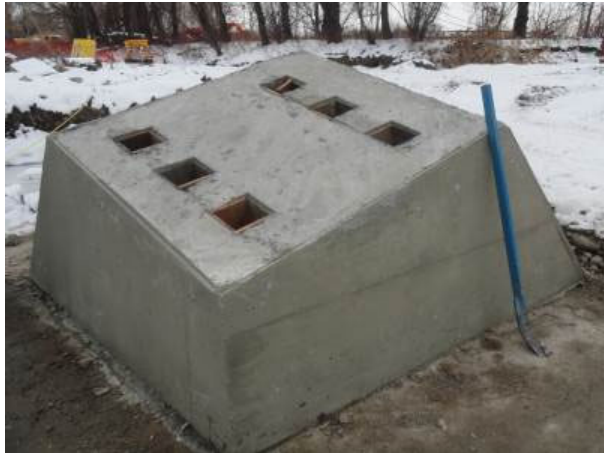
Fig. 14. Intermediate pier foundation.
