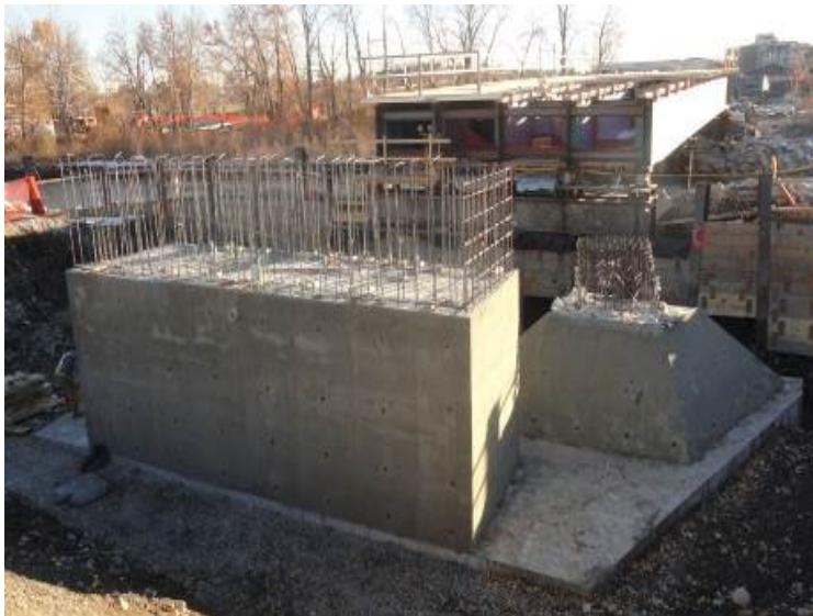
Fig. 13. Abutment pier foundation.
