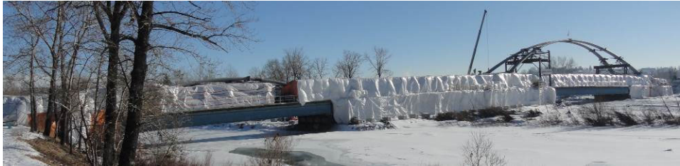
Fig. 19. Hoarding and heating of entire bridge deck during winter construction.
