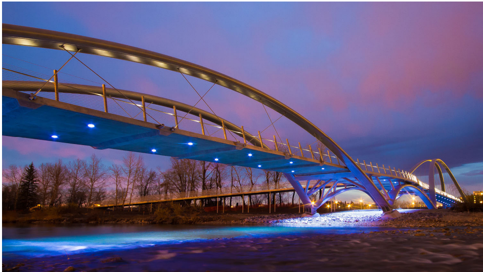
Fig. 20. Completed bridge and island access ramp with lighting.
