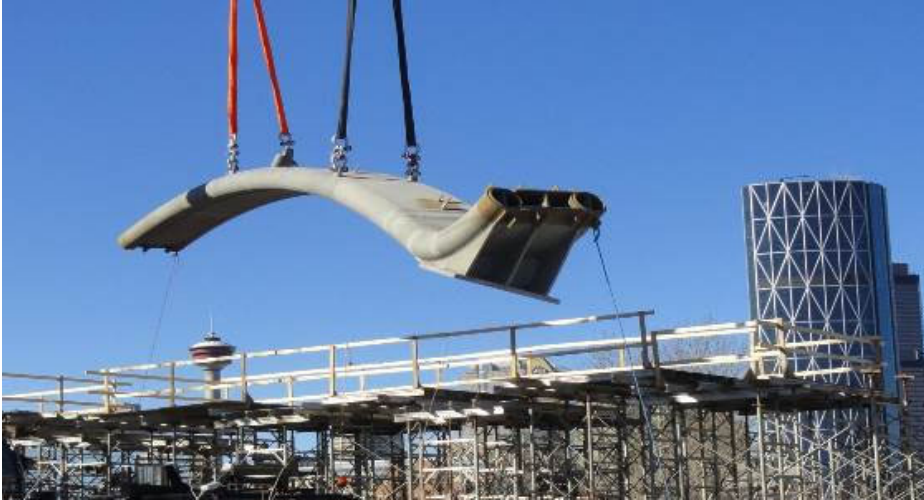
Fig. 7. Erection of centre arch segment.
