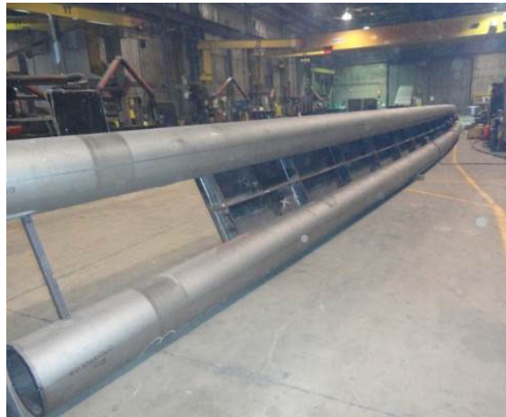
Fig. 4. Arch rib fabrication.
