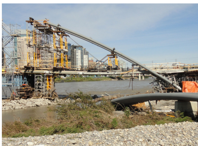
Fig. 17. Deck deflection after flooding.
