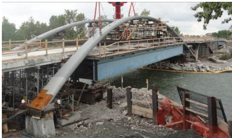
Fig. 9. North arches erected.
