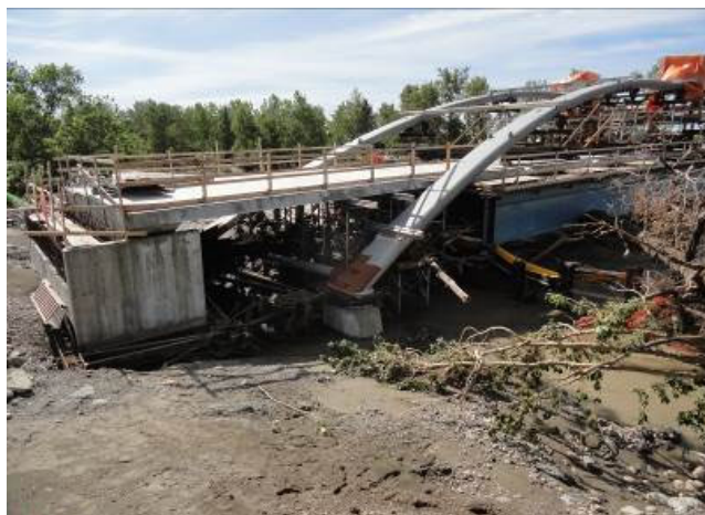
Fig. 16. Flood debris under north end.
