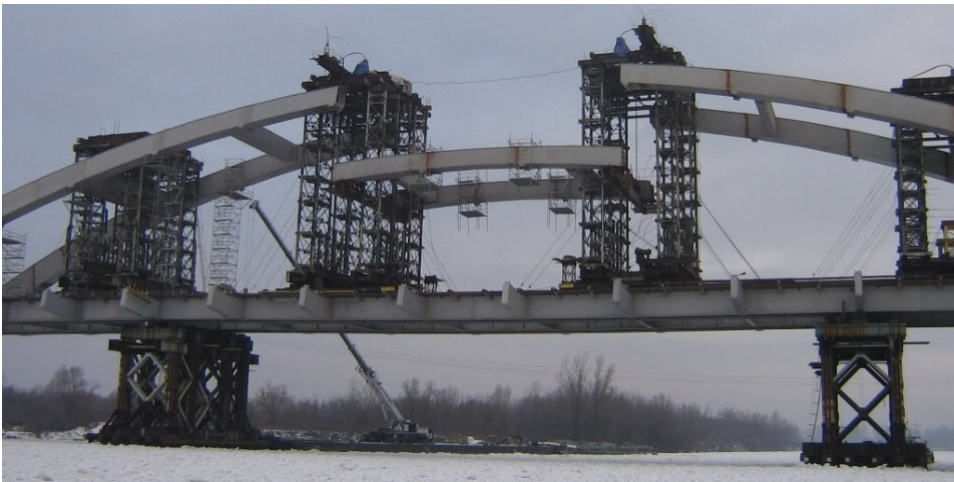
Fig. 14. Lifting of the last arch element.
