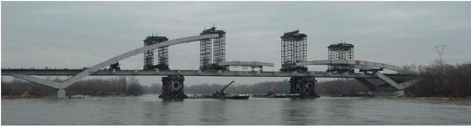
Fig. 13. All the arch elements ready for lifting and rotating.
