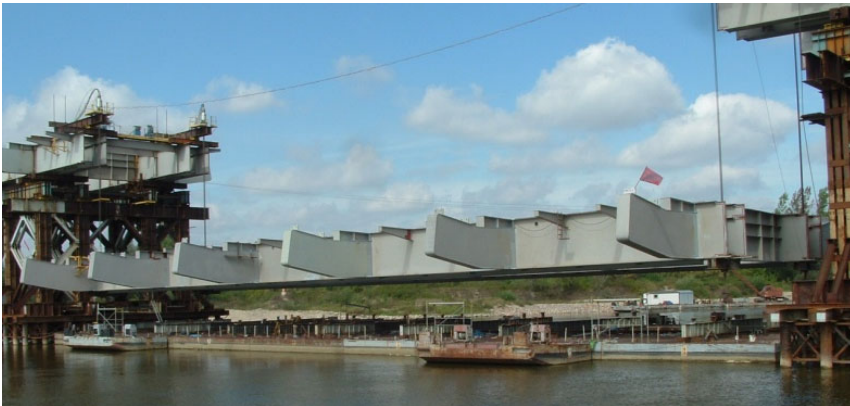
Fig. 9. Deck assembly in the river part.
