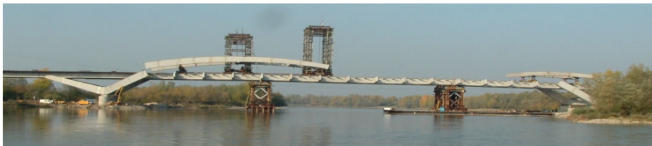
Fig. 12. Sliding of the first arch element.
