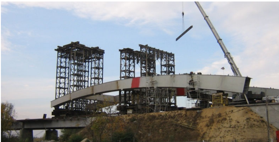
Fig. 11. The first arch element on the assembly site on the embankment behind the abutment.
