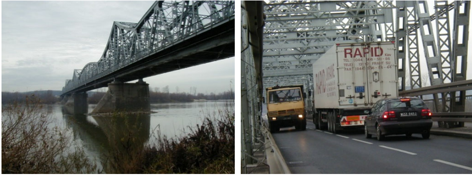
Fig. 2. The old bridge traffic jam.
