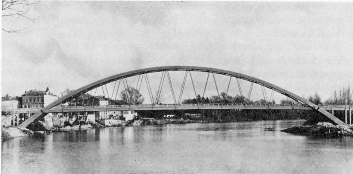
Fig.1. The Castelmoron Bridge built in France in 1933 i . Span 154 m.
