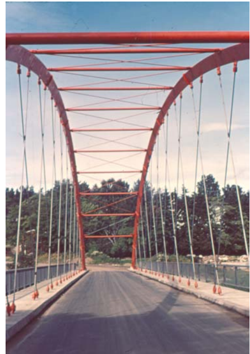
Fig. 3. Network arch at Steinkjer, Norway
