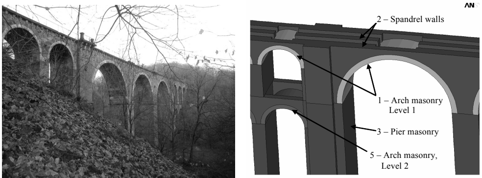
Figure 3: Masonry arch bridge (left), material areas (right)
