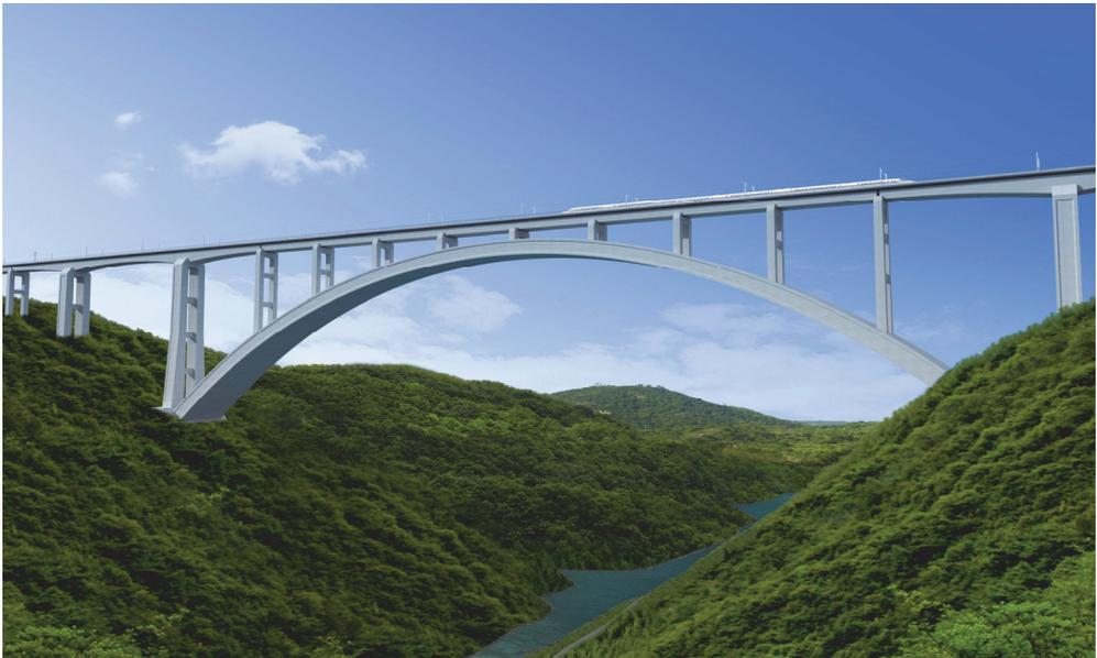
Figure 6: Rendering of deck concrete single box arch
