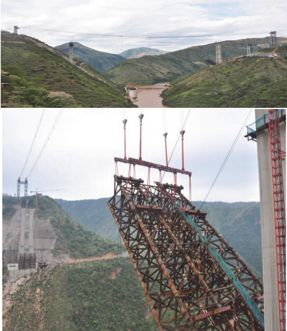
Figure 18: Erection of steel tubular truss
