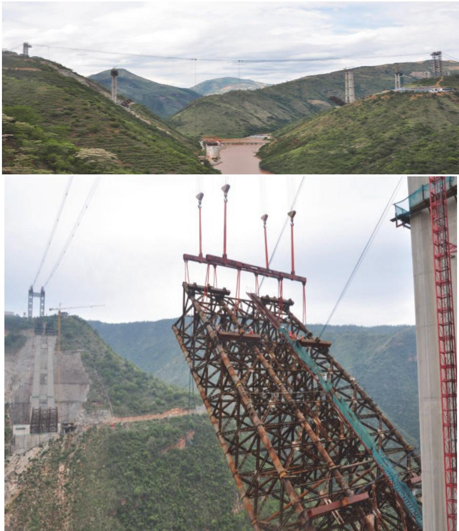
Figure 18: Erection of steel tubular truss
