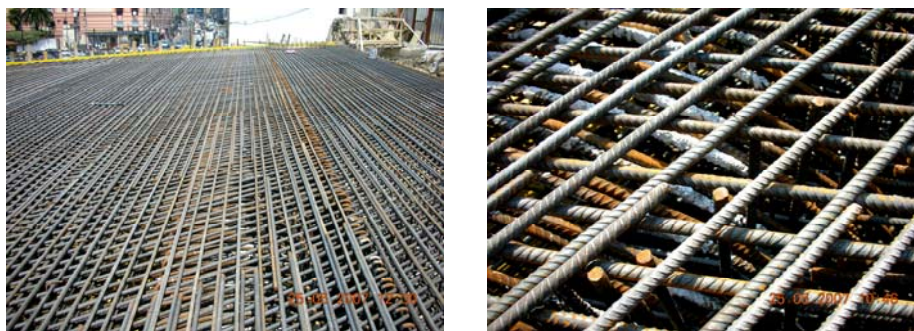
Figure 4 : The deck heavy reinforcement
