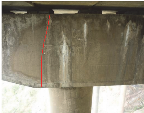
Figure 6: Vertical Crack on the Bent-cap (2012)
