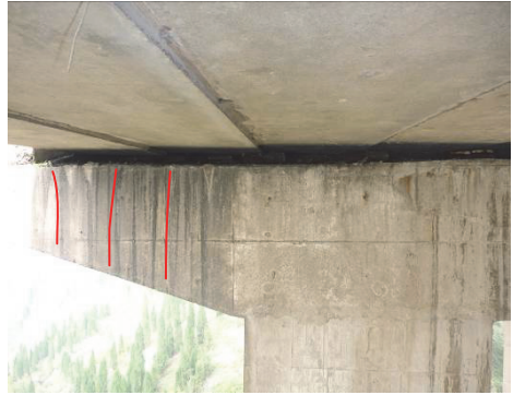
Figure 5: Vertical Cracks on the Bent-cap (2009)
