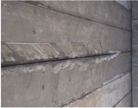
Figure 4: Water Penetration Between Slabs (2011)
