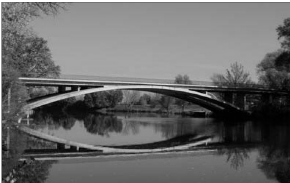
Figure 10. Bridge over Korana River in Karlovac (Rakovac)
