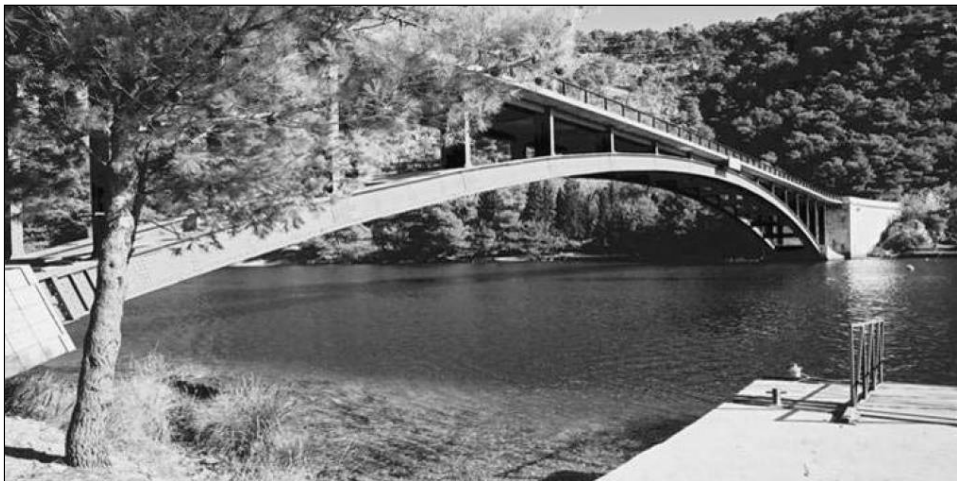
Figure 1: Bridge over Krka River in Skradin
