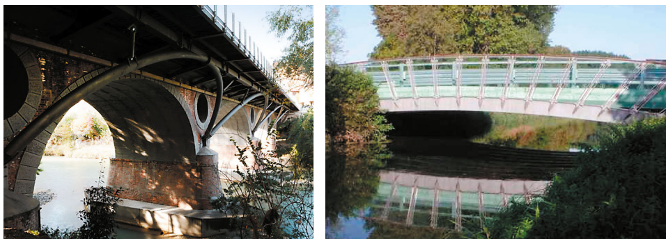
Fig. 11. E. Siviero: the bridge of Borgo Tossignano to the left; the bridge over the Tergola river in Villa del Conte (Padua) to the right.
