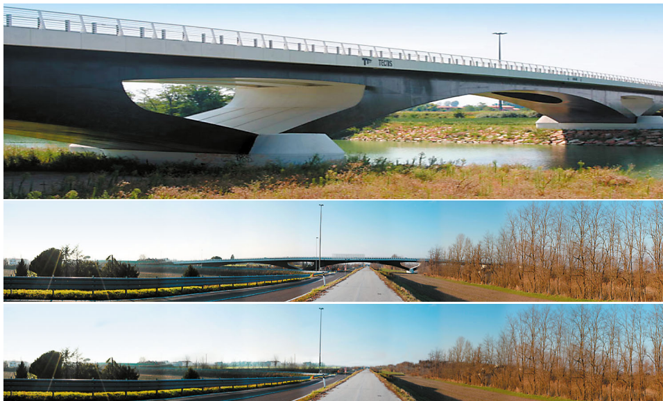
Fig. 10. E. Siviero. The bridge in San Donà di Piave, Venice. Perception of the bridge from the road.
