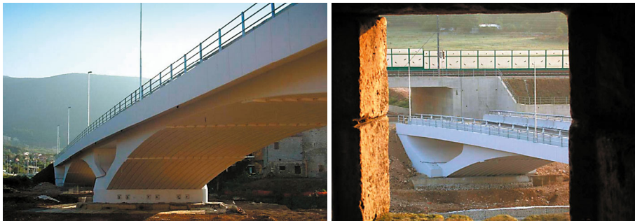
Fig. 9. E. Siviero, The bridge over the Sacco River.
