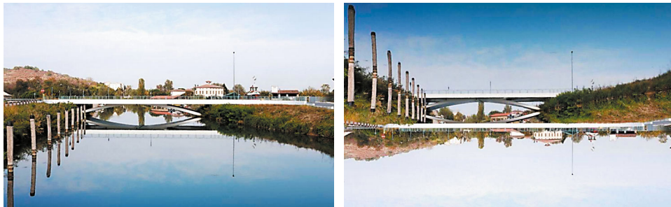
Fig. 6. E. Siviero, The bridge over the Battaglia Canal in the Province of Padua. They show the real situation (left) and the virtual one (right), with the bridge overturned. In both situations, the image of the bridge is the same, and the arch creates a virtual eye looking at you.
