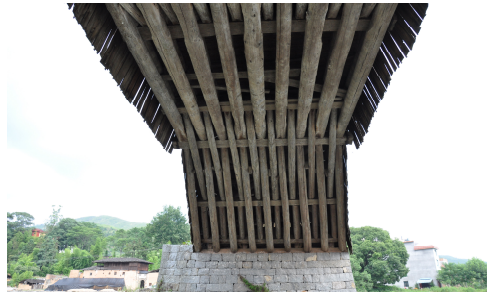
b) Up-view of a bridge
