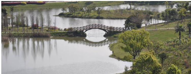
c) Bridge I in a bird view
