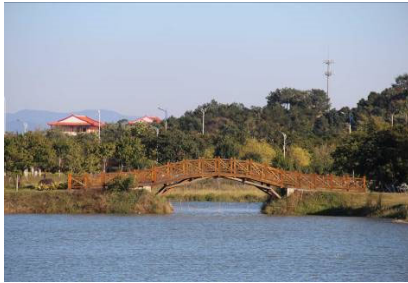
a) Bridge I in front view
