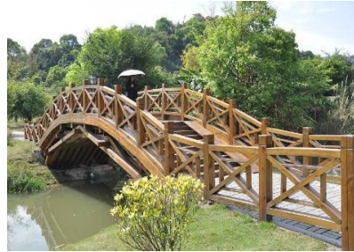
b) Bridge II in side view
