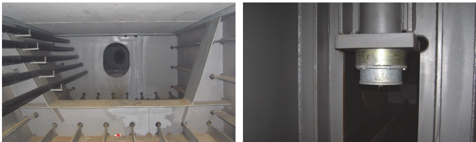
Figure 7: Inside view of the box girder (left) and passive anchorage of the hanger
