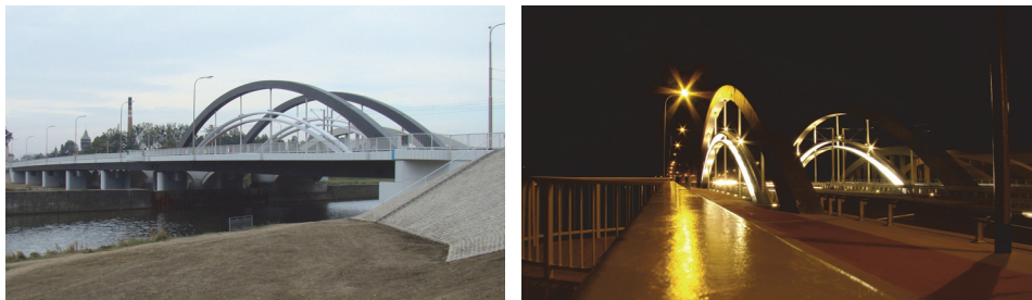
Figure 8: Overall day and night views of completed bridge
