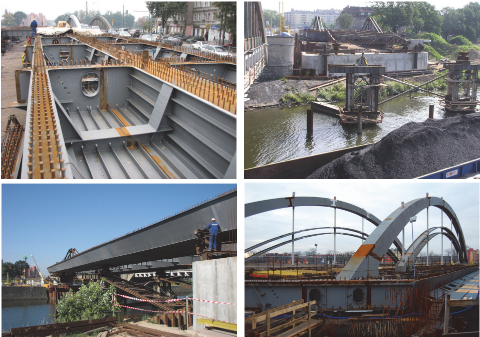
Figure 4: Assembly and launching of the eastern bridge superstructure
