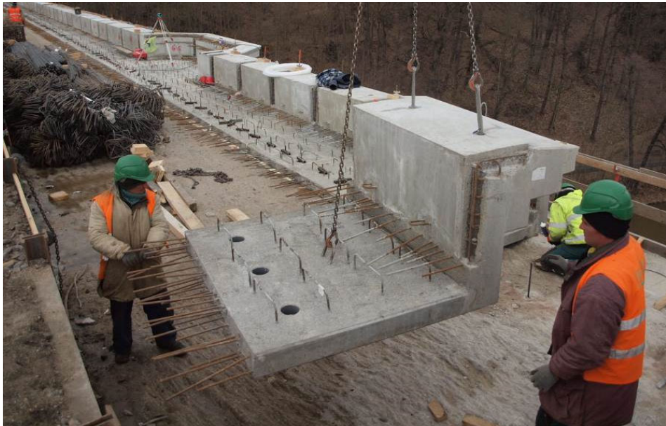
Fig. 6. Prefabricated elements during installation on bridge [4].
