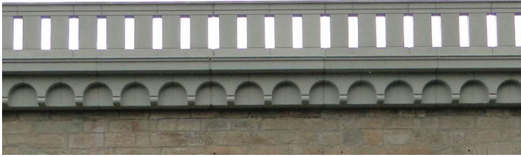
Fig. 7. Prefabricated elements after installation.
