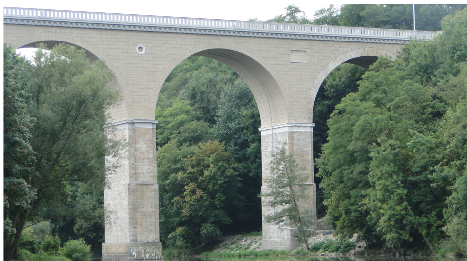
Fig. 9. General view of the bridge after modernisation – view on German side.
