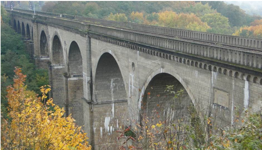
Fig. 2. General view of the bridge in 2011.
