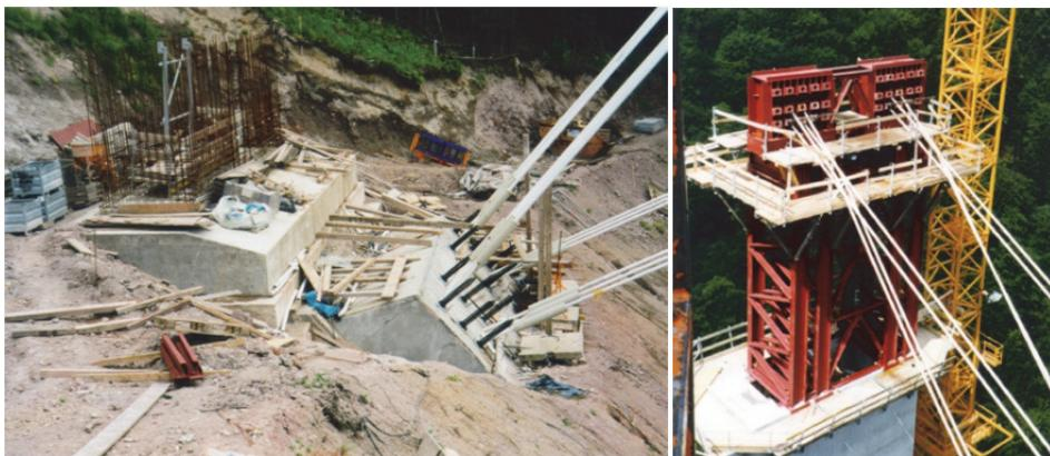
Figure 6: Anchoring of the cable stays at one of the footings
