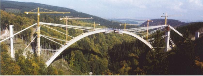
Figure 8: Arch just before the two halves were joined
