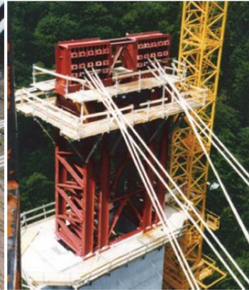
Figure 7: Temporary pylon on pier top of pier at arch springing
