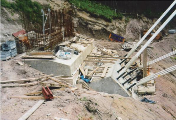
Figure 6: Anchoring of the cable stays at one of the footings
