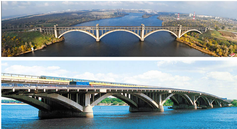
Fig. 8. Preobrazhensky Bridge in Zaporizhia on the top [10] and Metro Bridge in Kiev below [11]
