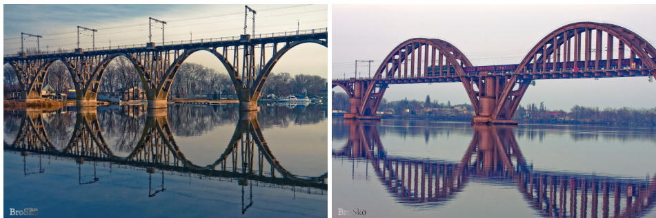
Fig. 7. Merefa- Kherson railroad bridge [9].
