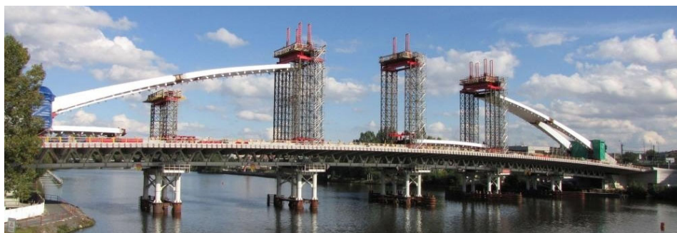
Fig. 10. Assembly of the outer edge parts.
