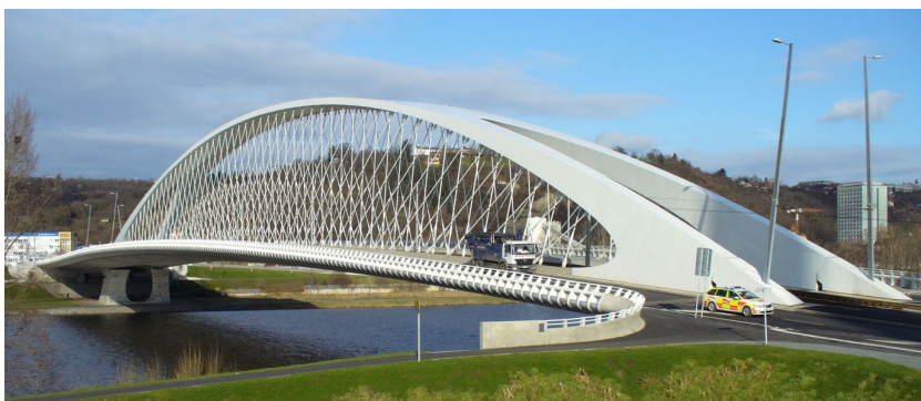
Fig. 1. View of the bridge.
