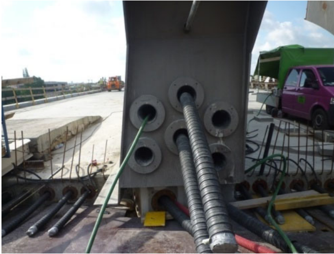
Fig. 4. Longitudinal prestress of the bridge slab.
