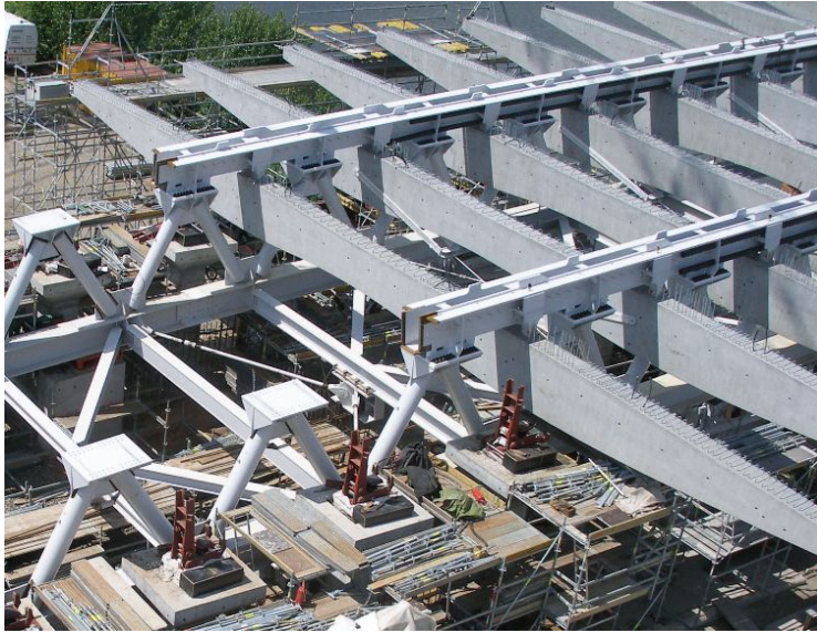
Fig. 8. Incremental launching of the temporary truss structure with cross-beams.
