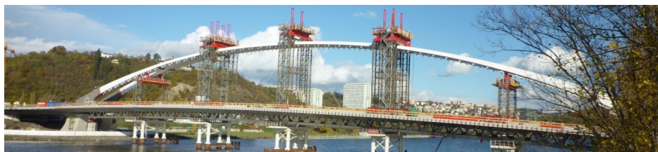
Fig. 11. Assembly of the central part of the arch.
