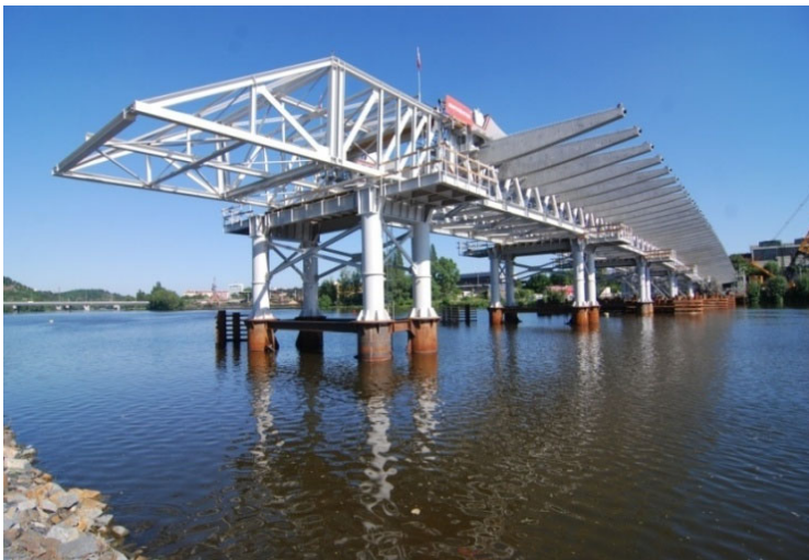
Fig. 9. Incremental launching of the temporary truss structure with cross-beams.
