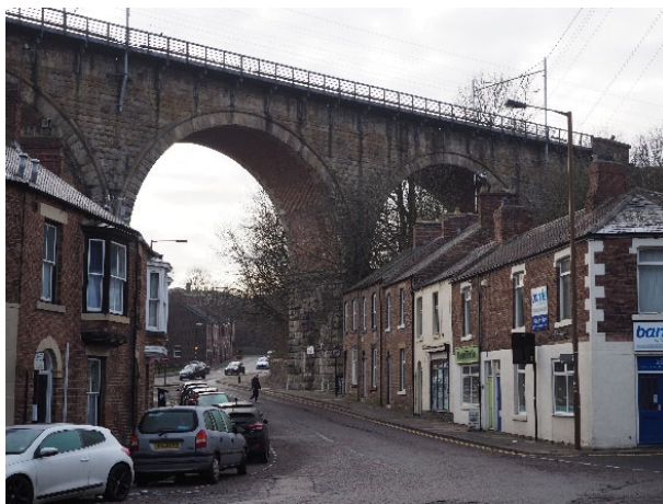
Fig. 10. Durham Viaduct – stone spandrels and voussoirs, brickwork arch barrel (Author's photograph).
