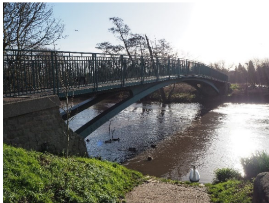
Fig. 14. Bridge over the Avon, Warwick, England (Author's photograph).
