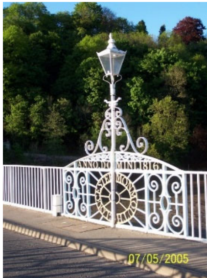
Fig. 6. River Wye Bridge, Chepstow, showing date of construction (Author's photograph).
