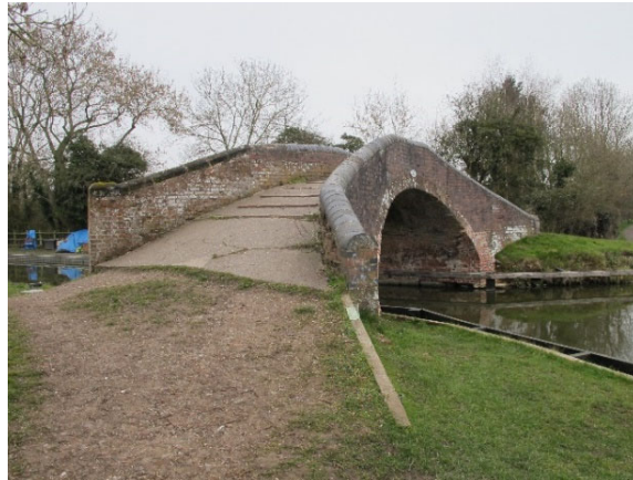
Fig. 8. Brickwork arch over the Grand Union Canal, Rowington, Warwickshire, England (Author's photograph).
