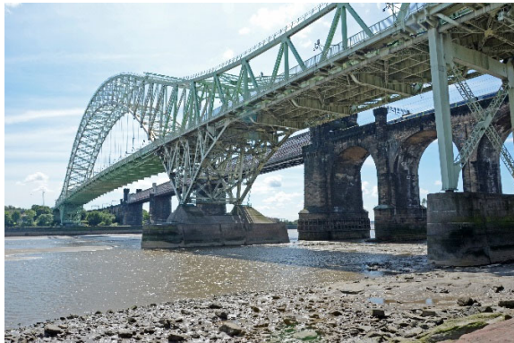
Fig. 13. Runcorn-Widnes Bridge over the River Mersey and the Manchester Ship Canal, England (Wikipedia).
