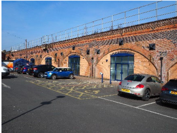
Fig. 9. Railway arches used as commercial premises, Leamington Spa, England (Author's photograph).
