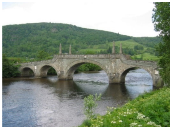
Fig. 4. Aberfeldy Bridge, built by General Wade over the River Tay, Scotland, 1733 (Wikipedia).
