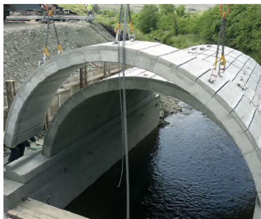
Fig. 16. Precast concrete arch unit being placed (Macrete, Co. Antrim, N.I.).
