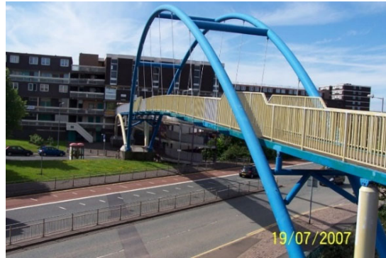
Fig. 15. Heath Town Footbridge, Wolverhampton, England (Author's photograph).
