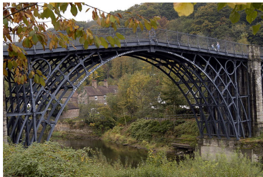
Fig. 5. The Iron Bridge, Shropshire, England (Wikipedia).
