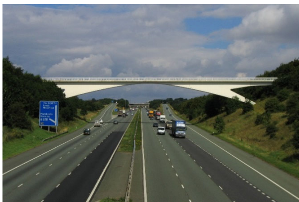
Fig. 12. Bridge over the M1, Barnsley, Yorkshire, England (Wikipedia).
