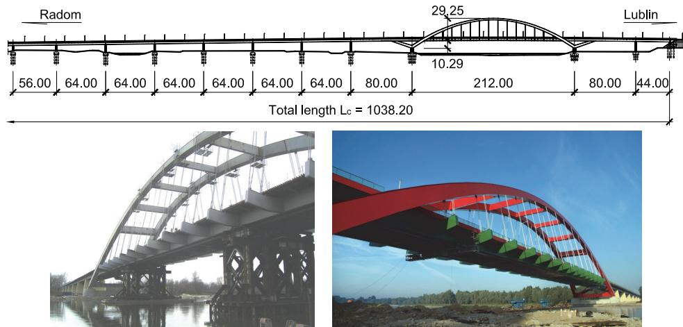
Figure 5: Bridge in Puławy: side view, view during construction and completed structure
