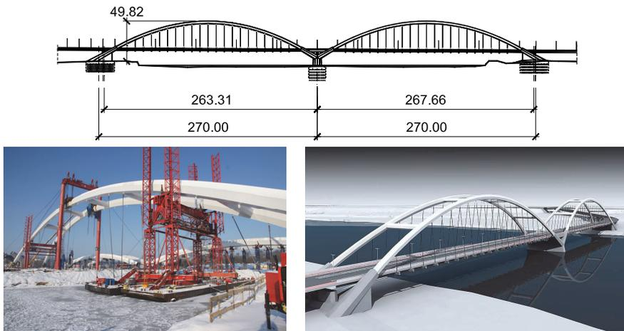
Figure 6: Side view, assembly of the arches (photo: K. Jędrzejewski – Strabag) and computer image of the bridge in Toruń [7]
