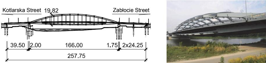
Figure 4: Side view and overall view of the Kotlarski Bridge in Cracow
