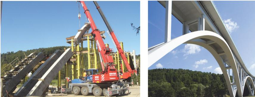
Figure 1: Bridge in Miłowka: side view, assembly of arch segments [1] and view of completed structure (photo: GDDKiA Katowice)
