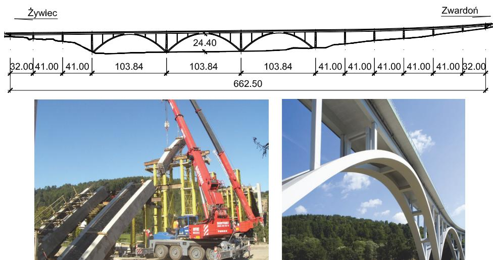
Figure 1: Bridge in Milówka: side view, assembly of arch segments [1] and view of completed structure (photo: GDDKiA Katowice)
