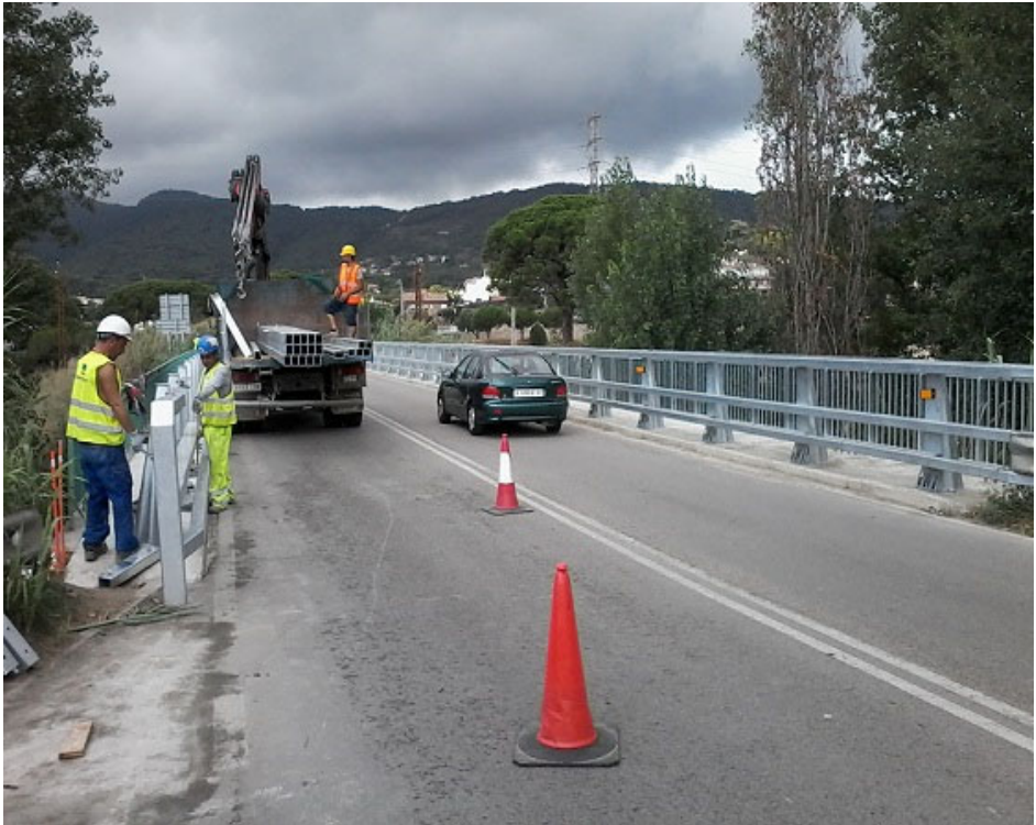
Fig. 17. Safety barrier installation.
