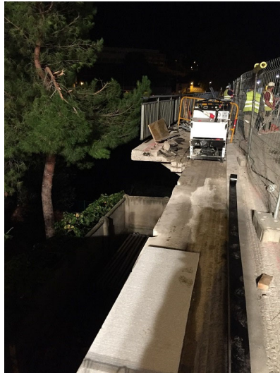
Fig. 5. Longitudinal base and neoprene bearing for the new precast slab deck.
