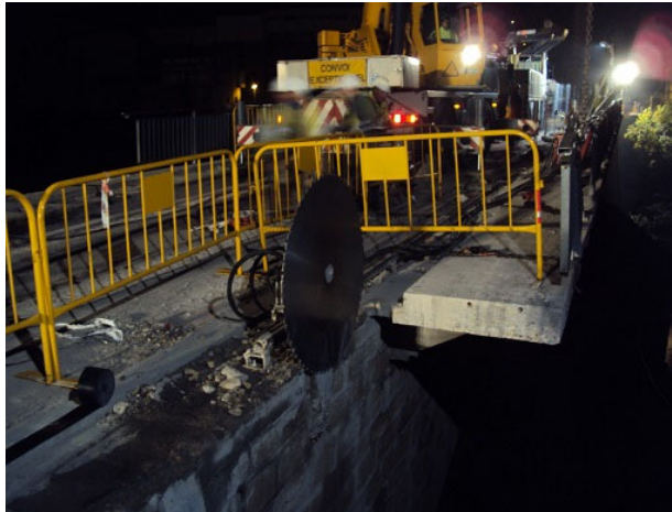
Fig. 6. Saw used to dismantle both cantilevers off of the main existing slab deck.
