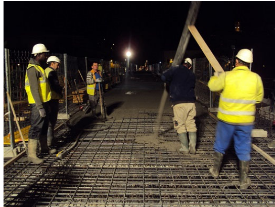
Fig. 8. Concrete pouring. In situ slab deck.
