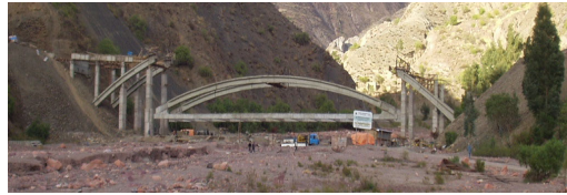
b) Bridge at final stage
