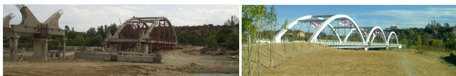
a) Bridge at assembling stage.
