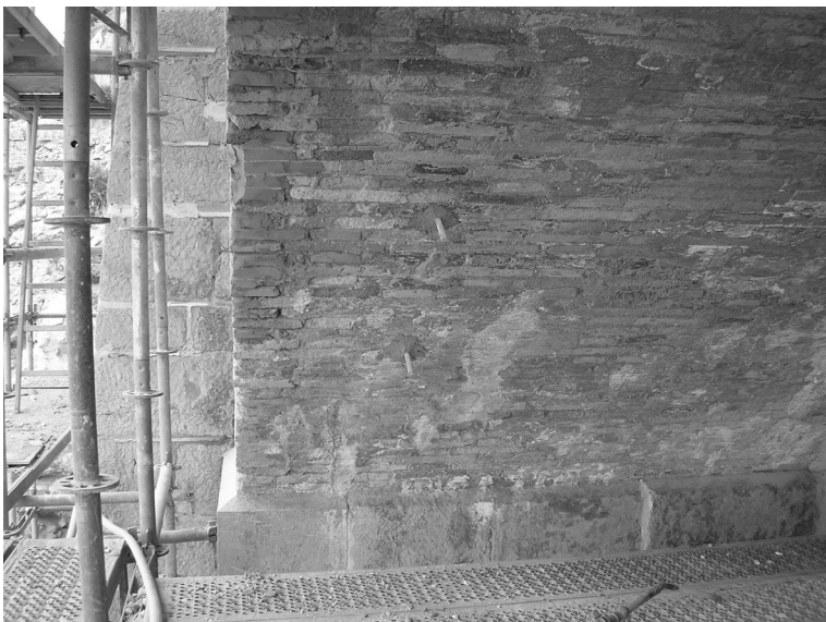
Photo 2: injection of arch extrados.
