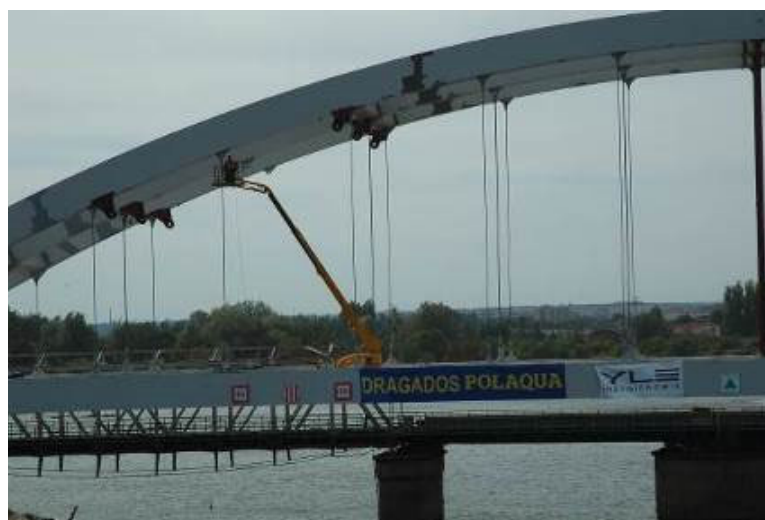
Fig. 16. Positioning of the remaining ropes.
