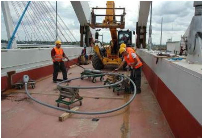
Fig. 11. Manual uncoiling of the ropes.
