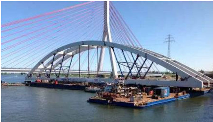
Fig. 14. Swimming in of the arch.
