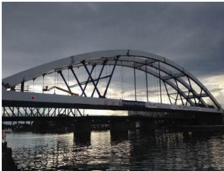
Fig. 15. Positioning of the ropes between temporary support of the arch.
