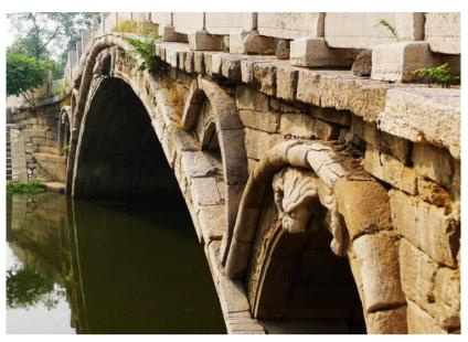
Fig. 7. The stones seriously weathered and eroded.
