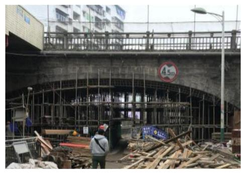
Fig. 10. Hooped with reinforcement concrete.
