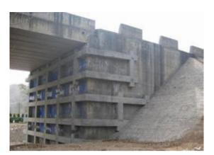
Fig. 11. Hooped by a frame beam with bolt grouting.
