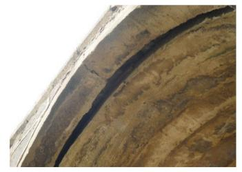
Fig. 2. Longitudinal cracks in the main arch ring.
