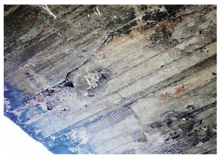
Fig.3. The transverse cracks in the spandrel arch ring.
