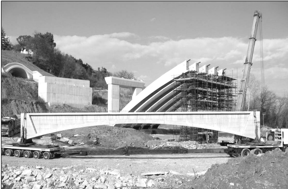
Figure 6 : Precast arch segments brought to the building site.
