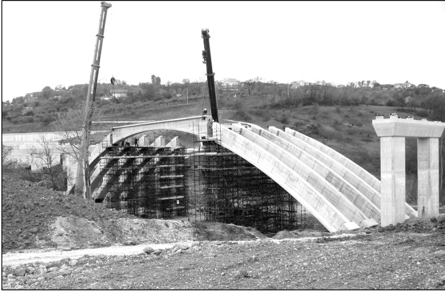
Figure 9 : Crane operated placement of the arch central elements
