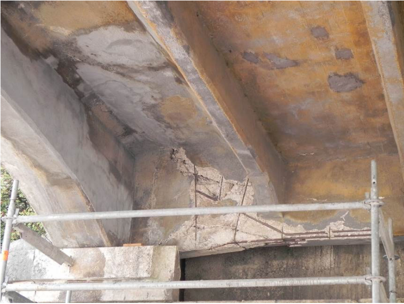
Fig. 5. First span: lateral view.
