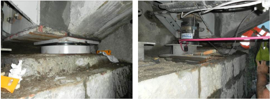
Fig. 15. New bearing and hydraulic jack.
