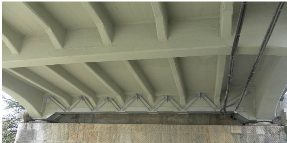
Fig. 13. Application of steel reinforcement.
