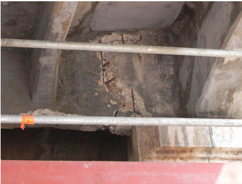
Fig. 6. First span: lateral view.
