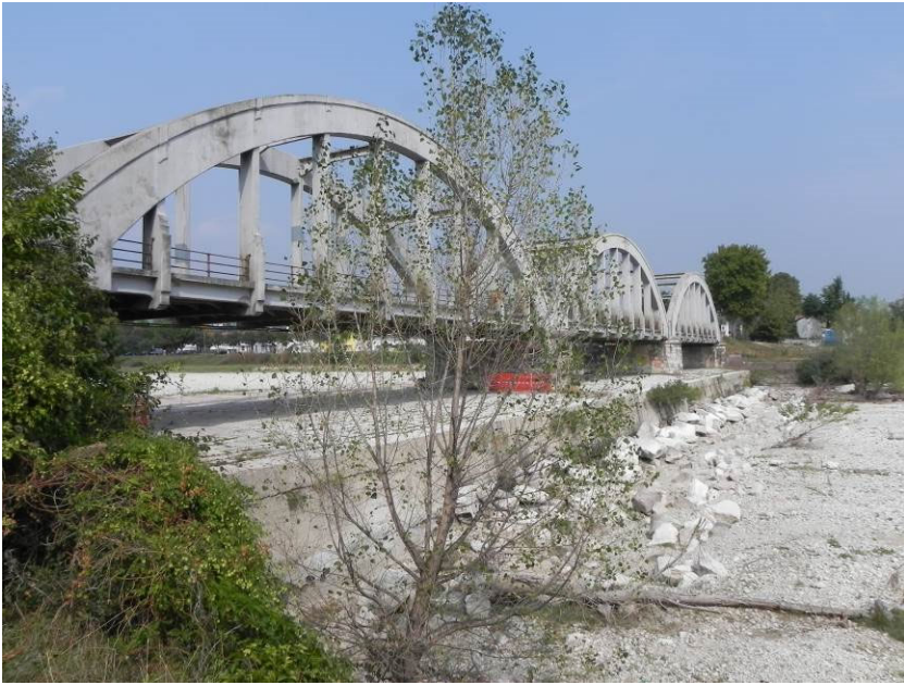
Fig. 1. Global picture of the bridge.
