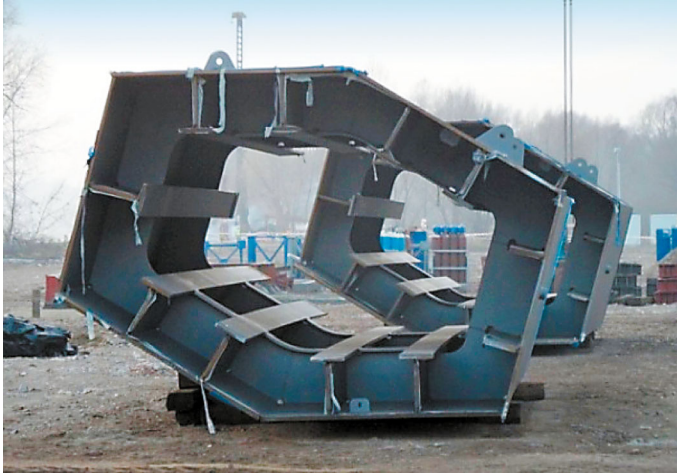
Fig. 11. Arch girder segment.
