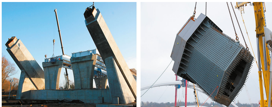
Fig. 20. Steel arch anchorage.
