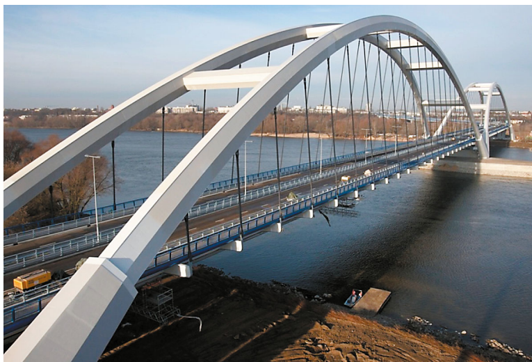
Fig. 1. View of Torun bridge (fot. A. Zakrzewski).
