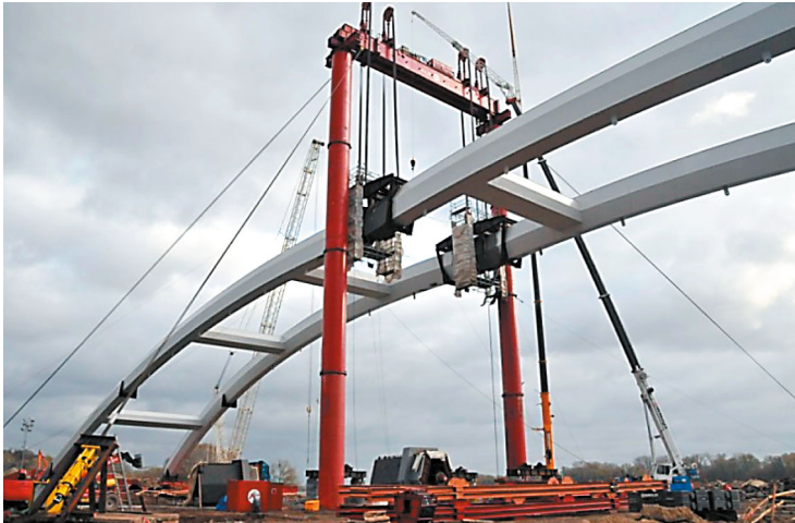
Fig. 14. Lifting tower – arch head joint.
