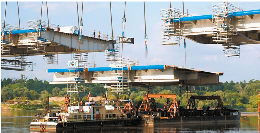
Fig. 17. Deck heave lifting.
