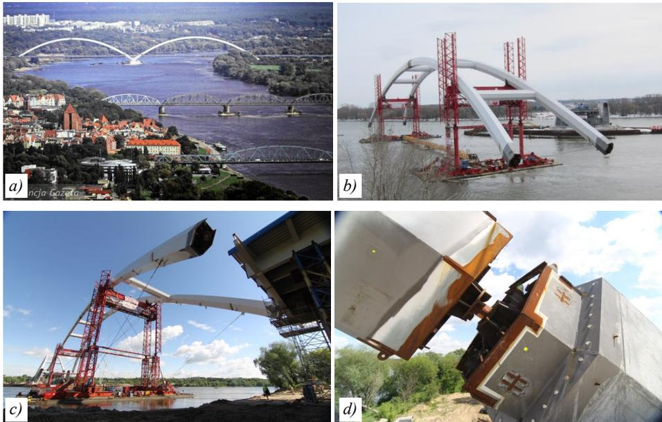
**Fig. 2.** a) Bridges of Torun; b) assembly of bay arch girders 13-15; c) assembly of bay arch girders 15-17; d) assembly table for placing an arch girder on a head section
