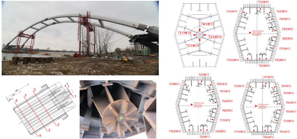
**Fig. 6.** General view of the structure after placing arches of a bay 13-15 on assembly tables; layout of cross-sections and strain gauge measuring points of a head section no. 13 (till the moment of bracing of bay part with supporting part of arches).
