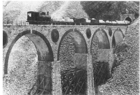
Figure 2: Pier propped up after failure in 1913
