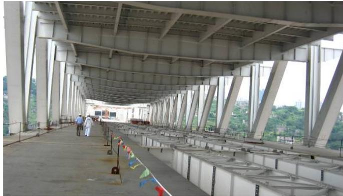
Figure 5 : Upper and lower decks of Main Bridge
