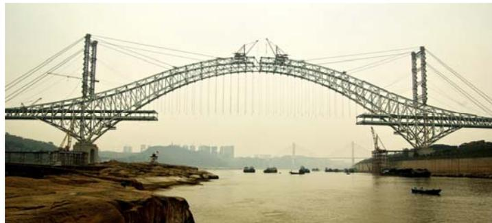
Figure 7 : Arch ribs before closure in mid span during construction
