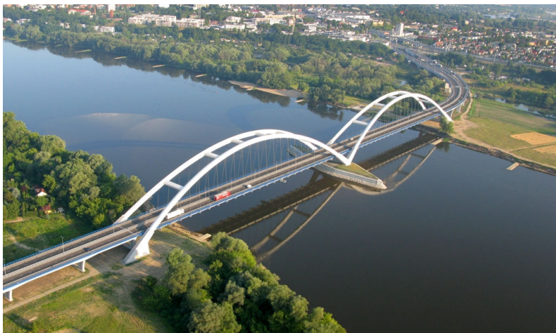
Fig. 1. View over the bridge in Toruń.
