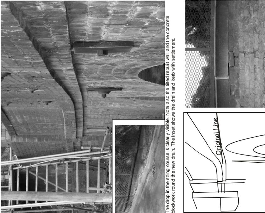
The drop in the string course is clearly visible. Note also the tiled rebuilt wall and the concrete blockwork round the new drain. The inset shows the drain and kerb with settlement.
