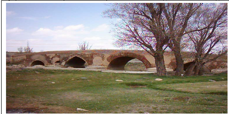
Figure 7: Picture of Abshineh Bridge, Hamadan
