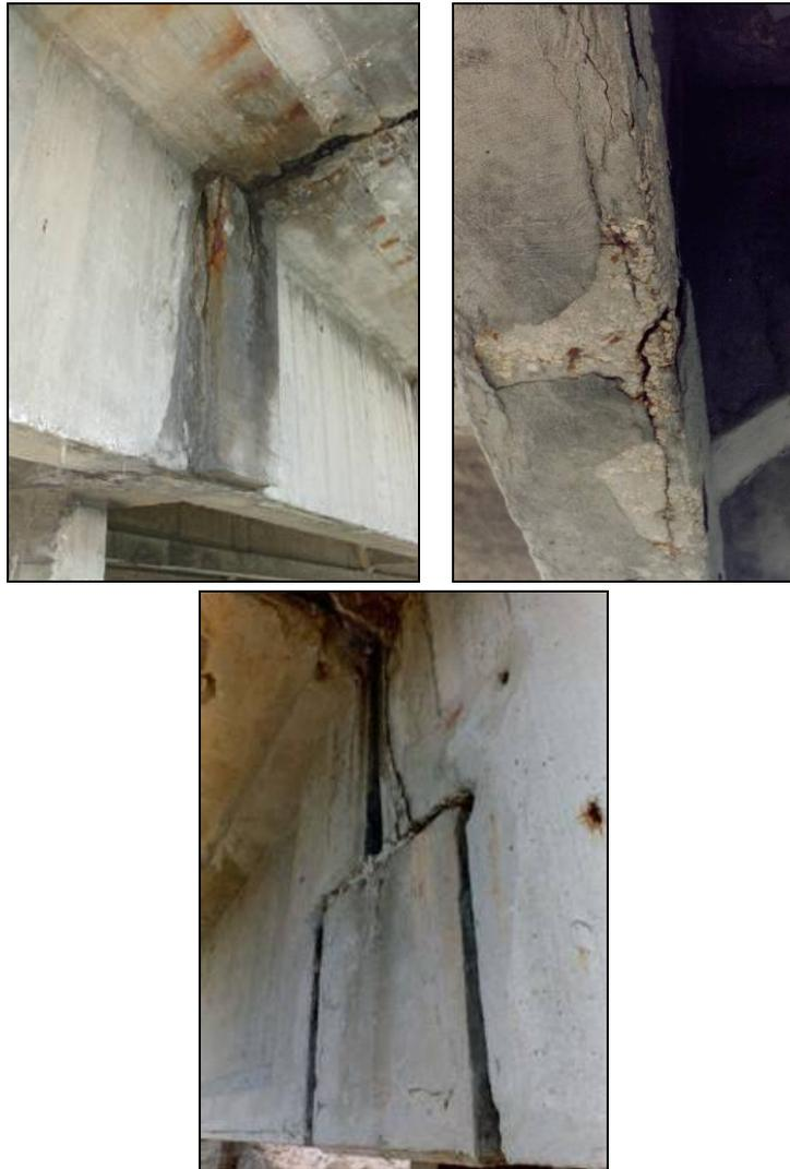
Figure 5 : Sibenik (left), Pag (center) and Krk (right) Bridges: deterioration of bridge superstructure
