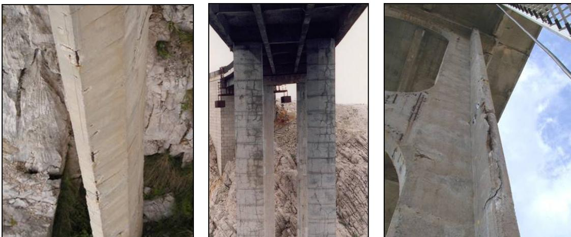
Figure 6 : Sibenik (left), Pag (center) and Krk (right) Bridges: deterioration of columns
