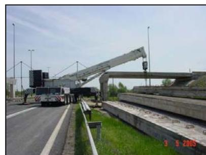
Figure 4 : Reconstruction of a severely deteriorated motorway overpass
