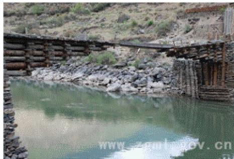
Figure 3: Structure of Flat Stacked Girder Arch Bridge of Muli in Sichuan Province, China.
