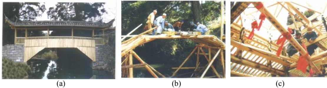
Figure 8: Shijin Bridge: (a) The Shijin Bridge, (b) Install the main arch rib, (c) Raising of the ridgepole
