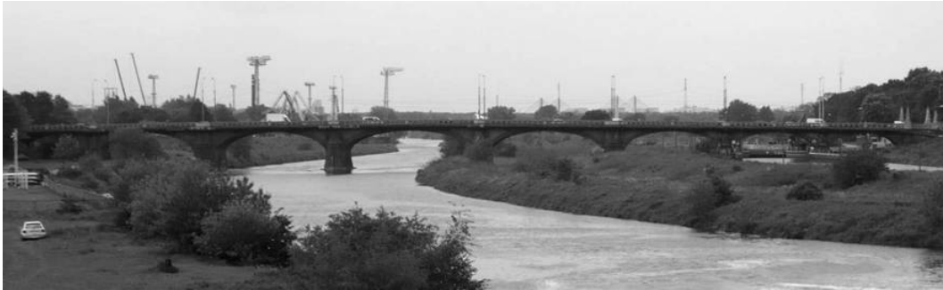
Figure 1 : The general view of the Osobowicki Bridge in Wrocław.
