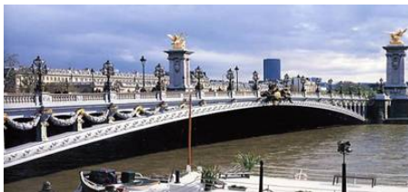
Figure 4 : Alexandra III Bridge
