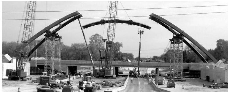
Figure 15: Erection of center rib with temporary towers
