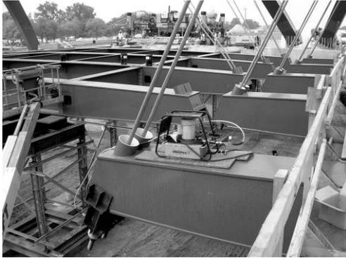
Figure 11: Hanger assembly – two strands
