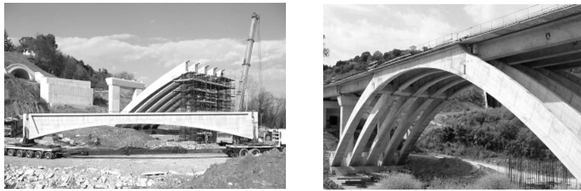
Figure 11 : Mazzocco Bridge, Pescara, designed by Mario Paolo Petrangeli, 70 meters span, 2007
