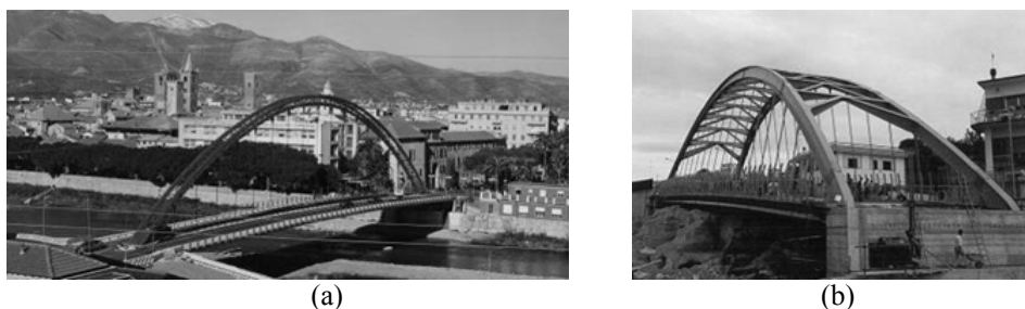
Figure 8 : (a) Steel arch bridge in Albenga, designed by Luca Romano, 100 m, 1996, (b) Steel arch bridge in Pozzuoli designed by Luca Romano and Pierangelo Pistoletti, 58 m, 1997
