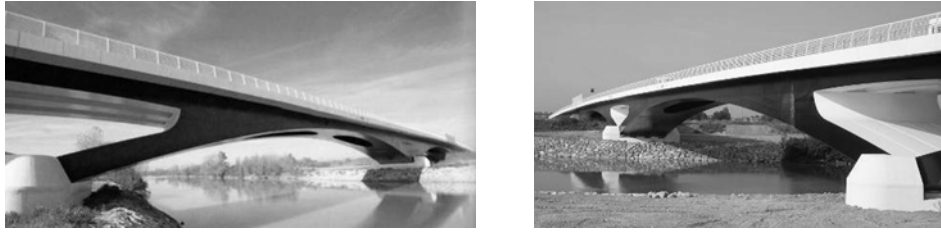
Figure 9: San Donà Bridge, Venice, designed by B. Briseghella, E. Siviero, T. Zordan, 500 meters (L = 4x100 m), 2008
