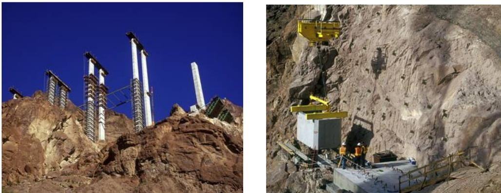
Figure 13 : Precast Column Erection
