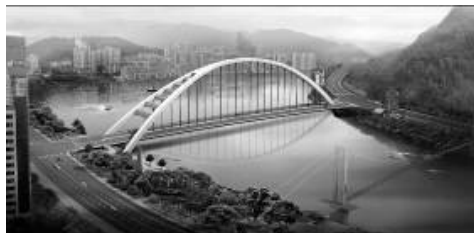
Figure 1 : View of the bridge with three ribs
