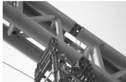
Figure 11: Connection of Arch Rib Segment
