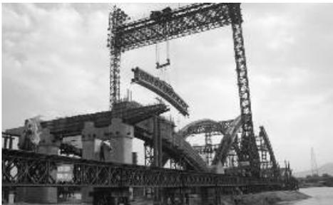
Figure 10: Temporary Bridge and Gantry Crane
