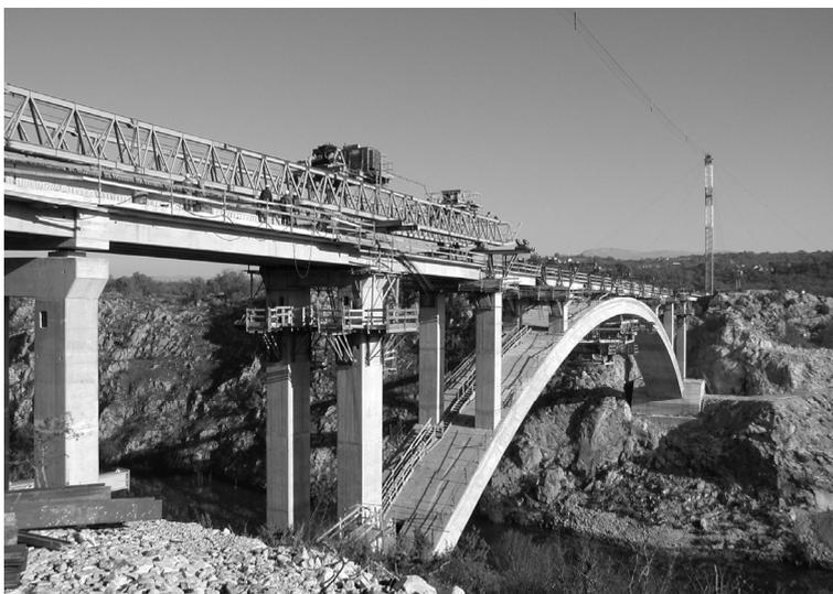
Figure 5: Superstructure construction
